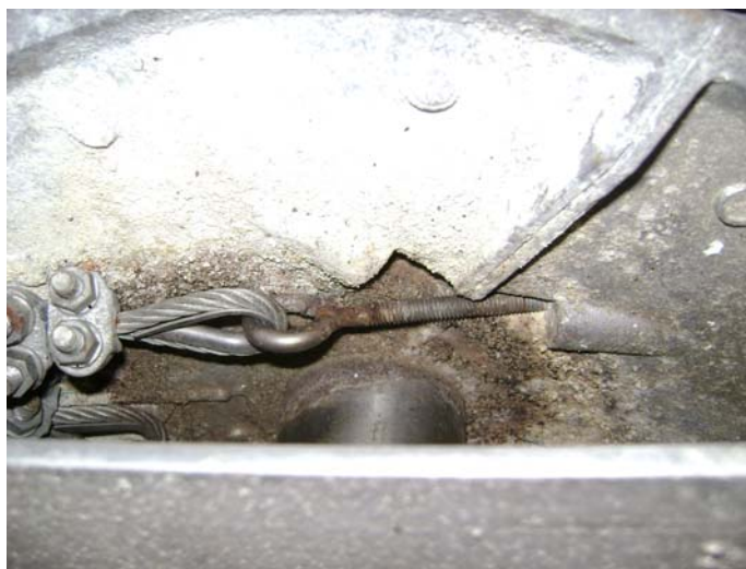
Steering quadrant bolt backing out.
