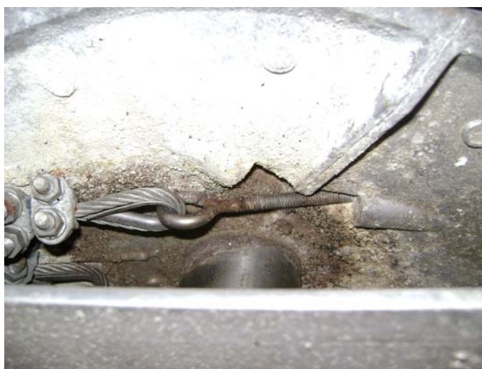
Steering quadrant bolt backing out.
